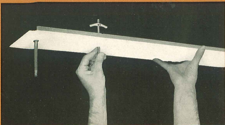
To install flush mounted Royal fasten cover plate to ceiling with toggle bolt.
